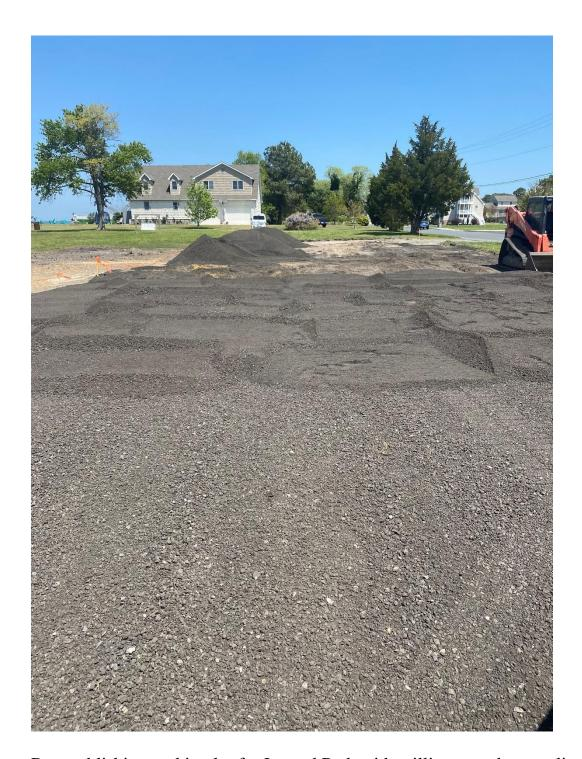
Re-establishing parking lot for Lenard Park with millings as a base, split-rail fence. Topsoil and seeding will be installed outside the parking area.
